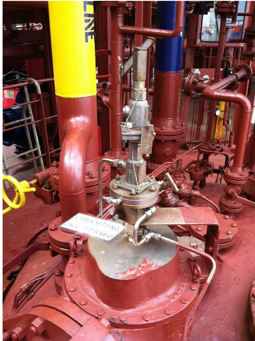
Figure 11-9 Relief valves stacked correctly, typical LPG set-up
