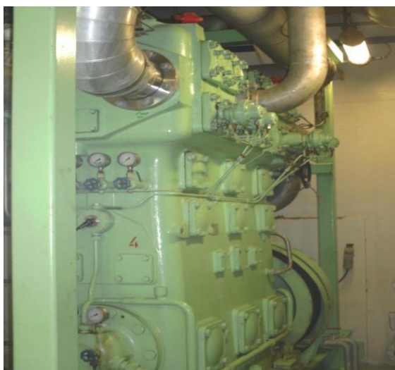
Figure 11-12 Three-stage cargo compressor on an LPG gas carrier
