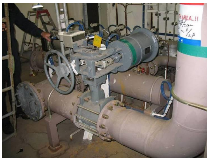
Figure 14-5 Example of second fail-closed shutoff valve installed in series with the MGV in the boiler hood or gas room
