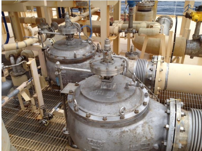
Figure 11-6 Cargo relief valves
