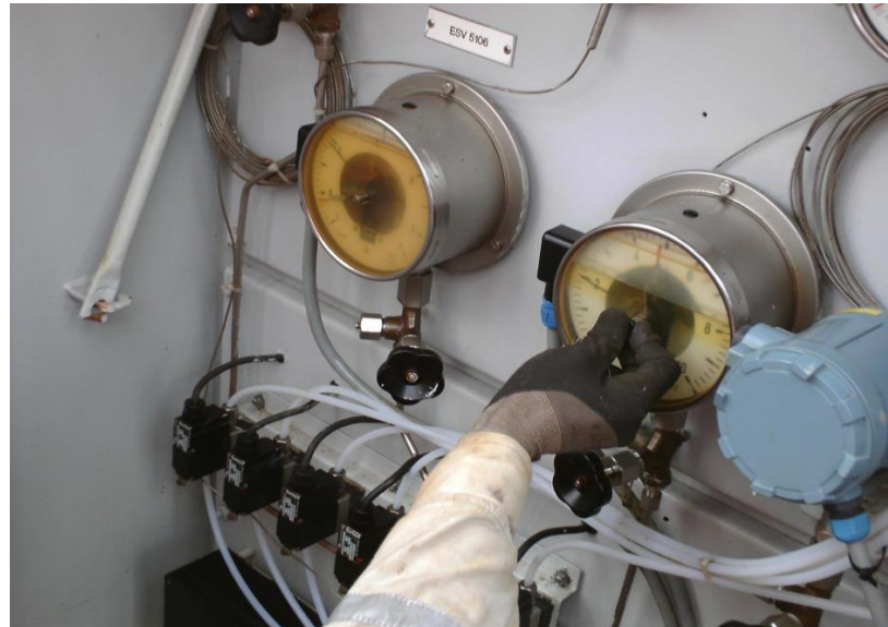
Figure 9-20 Testing of the high/low pressure alarm using a special handle
