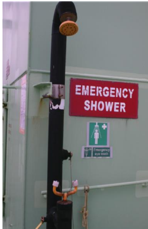
Figure 5-1 Suitably marked decontamination shower and eye wash station
