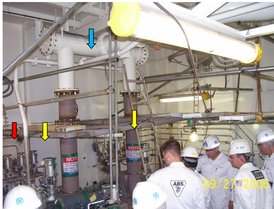
Figure 14-7 Fail-open vent valves
