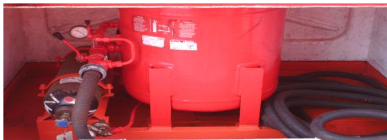
Figure 7-3 Dry chemical powder fire extinguishing system
