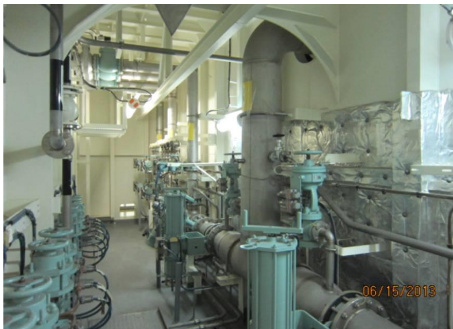
Figure 14-9 Gas utilization room on LNG gas carrier
