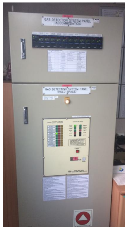
Figure 9-6 Combined suction (holds/un-manned spaces)/electronic (accommodations/manned spaces) fixed gas detection system
