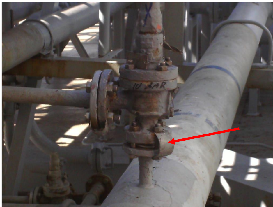
Figure 11-10 Electrically bonded relief valve
