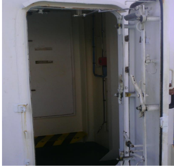
Figure 5-4 Air lock (note the two steel doors)
