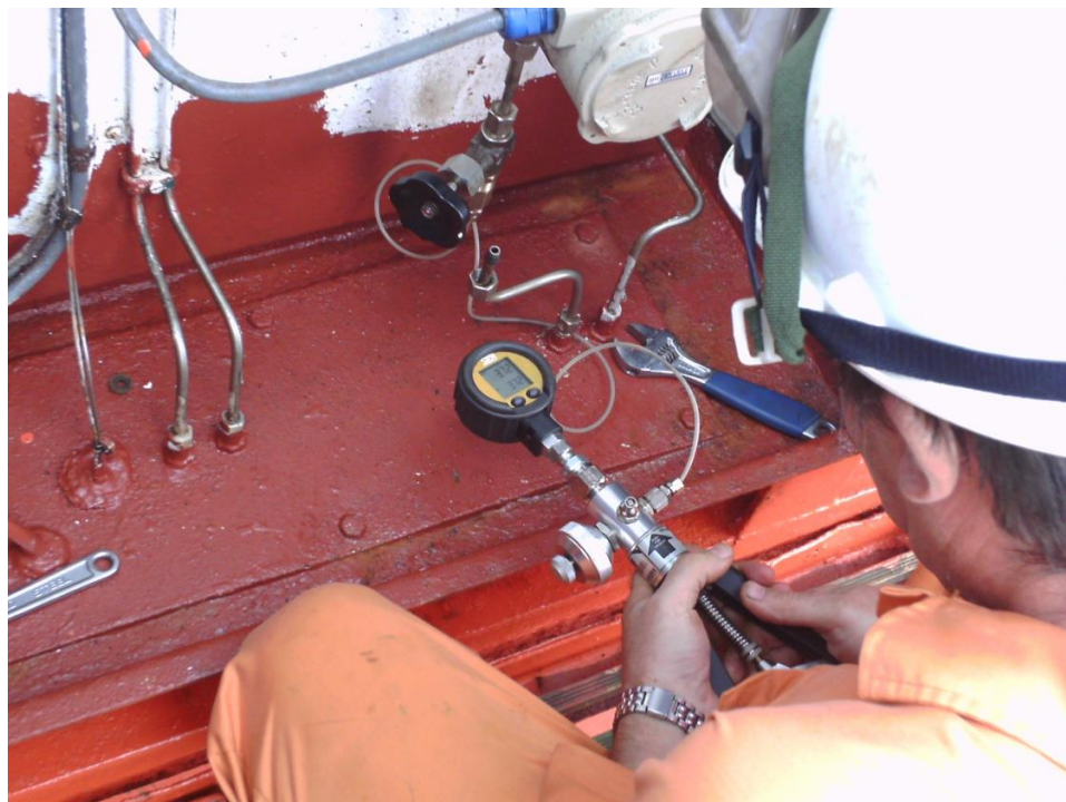
Figure 9-21 Testing of the high/low pressure alarm using a hand pump
