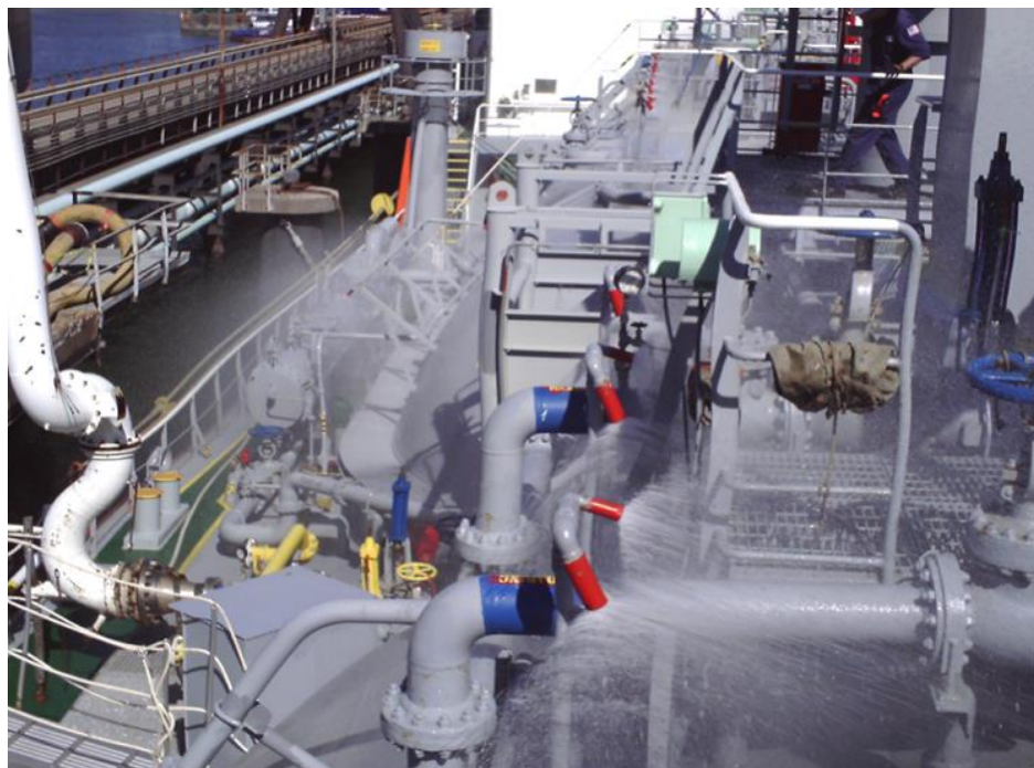
Figure 7-1 Activated deck water spray system (manifold)
