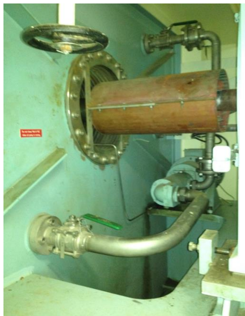
Figure 11-14 Lubricated bulkhead shaft seal passing through the gas tight bulkhead on an LNG gas carrier
