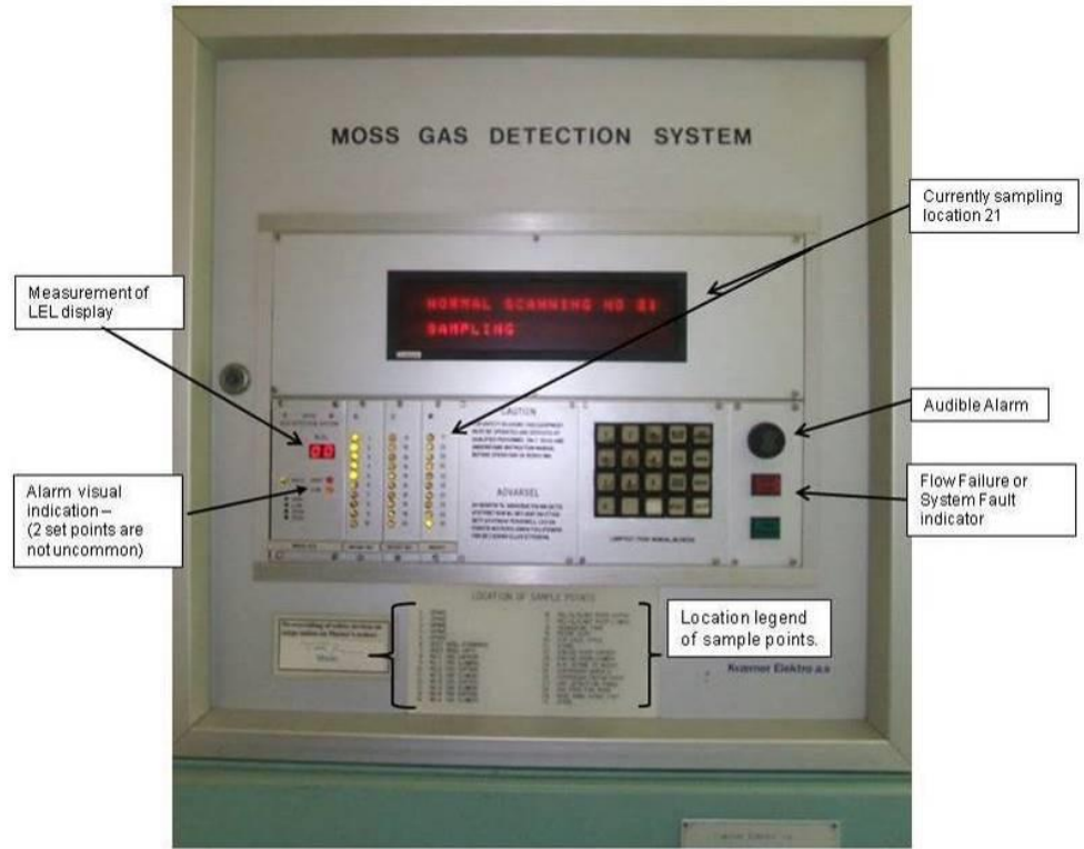
Figure 9-1 Gas detection system
