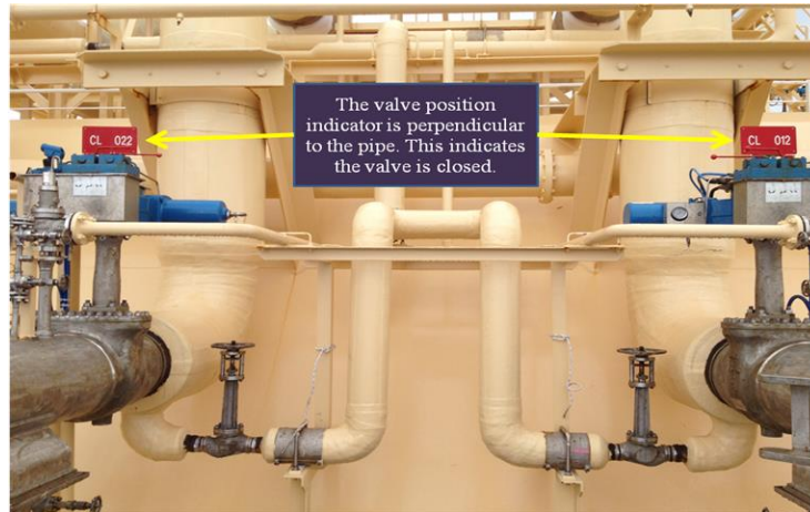
Figure 11-5 Valves position perpendicular to the pipe
