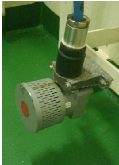
Figure 9-8 Electronic sensor sample point
