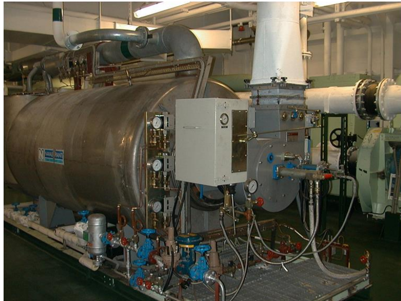
Figure 12-1 IGS on a gas carrier
